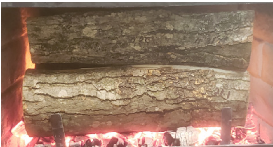
Figure 30: Low-fire load in firebox
